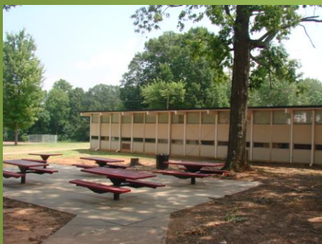
One of 2 Courtyards
