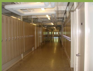
Locker lined Hallways
